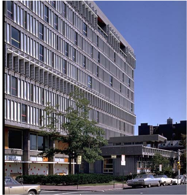
Corbu comes to Cambridge: Harvard's Holyoke Center by Sert, Jackson & Gourley, 1960-64. Photo by G. E. Kidder Smith, MIT Rotch Visual Collections. Along with this tribute to Le Corbusier's Unité, Sert also brought the master to Harvard to design the Carpenter Center, his only building in the United States.
