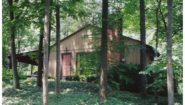
Cummins House, entrance front on South Brent Avenue
