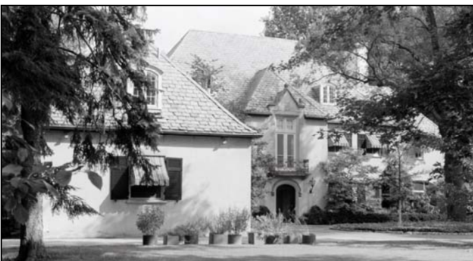
Lida Wallace Smith House, 9 St. Andrews Dr., Ladue, built in 1929, from the northeast.
