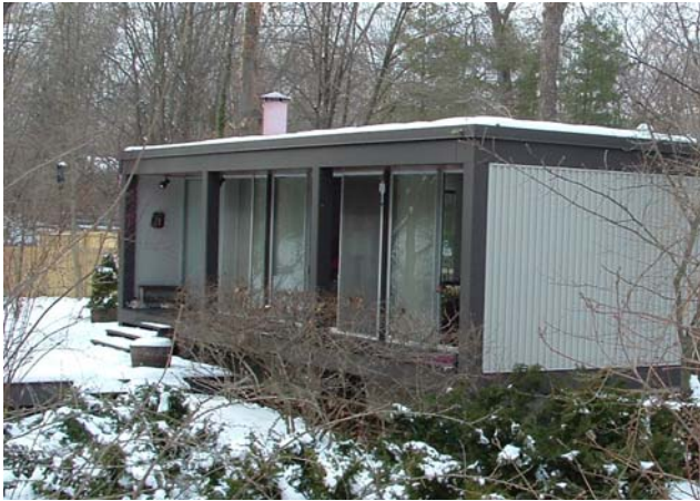
Robert Schutt House, south elevation toward creek
