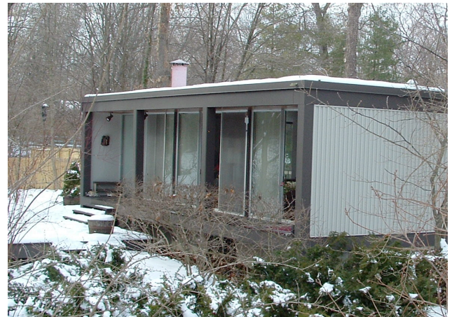
Robert Schutt House, south elevation toward creek
