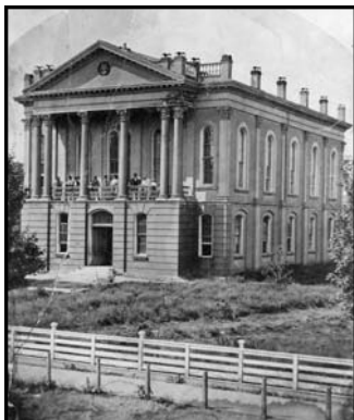
Madison County Courthouse, Edwardsville, Illinois. Courtesy of the Madison County Historical Society (IL). Demolished 1914.
