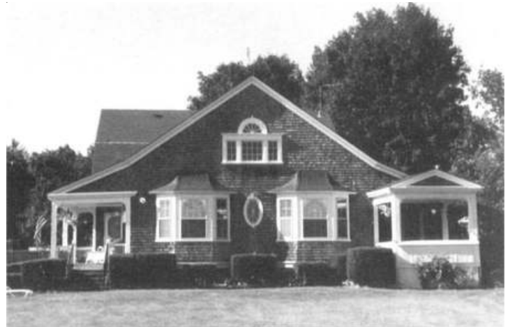
The Shoreby Hill Club, c. 1898, 75 Conanicus Avenue. Built as the Shoreby Hill Club, this building was moved to its present site in 1911 and became the Jamestown Casino. It is now a private residence.
