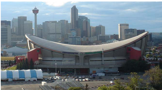
Olympic Saddledome (now Pengrowth Saddledome), Calgary, Canada, 1983, Graham McCourt Architects
