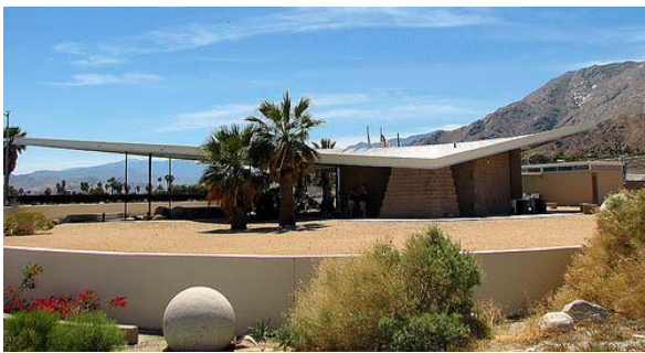
The Tramway Gas Station, now the visitors center for Palm Springs, California, designed in 1965 by Albert Frey
