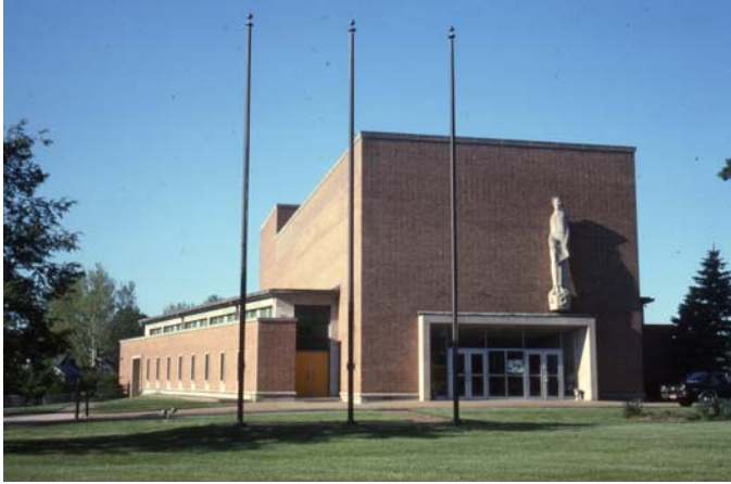
Joseph Murphy, St. Ann of Normandy Catholic Church , 7530 Natural Bridge Road, 1952; façade sculpture by Hilles Arnold
