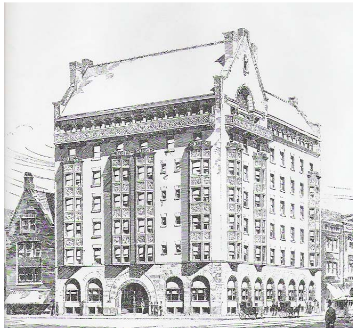
Drawing labeled "Hotel St. Nicholas, St. Louis, MO, Adler & Sullivan, Chas. K. Ramsey, Associated Architects" Published in American Architect and Building News. October 5, 1895 (Vol. L, No. 1032). Previously published in the St. Louis Post-Dispatch, November 13, 1892.
