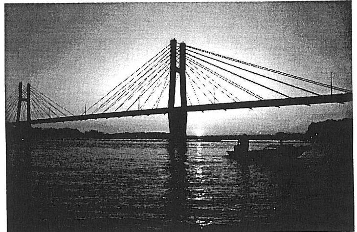
The New Quincy Bridge
