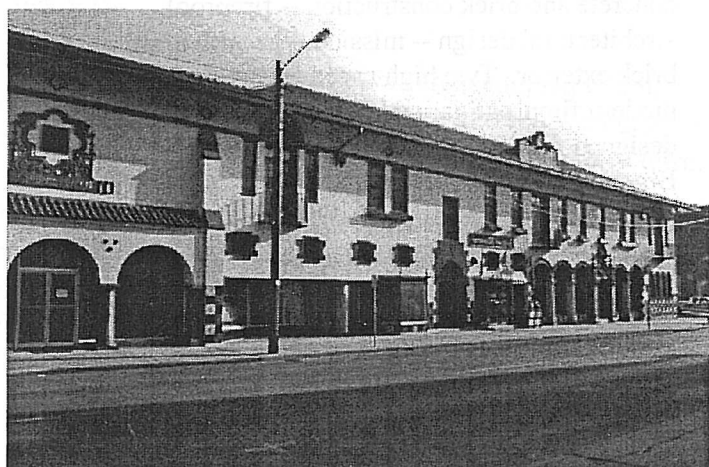
Southeast Missouriian building, Cape Girardeau, 1925, Tom P. Barnett. Photo by Bonnie Stepenoff
