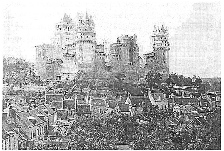
An image from the Russell Sturgis Collection: Pierrefonds, in the Forest of Compeigne north of Paris, built 1396-1406 for Louis of Orleans and restored 1858-1885 by Emmanuel Viollet-le-Duc. These photos apparently date from the mid-1860s, when the exterior restoration of the donjon had been completed but before much had been done on the outer walls. Scaffolding can be seen in the background.
