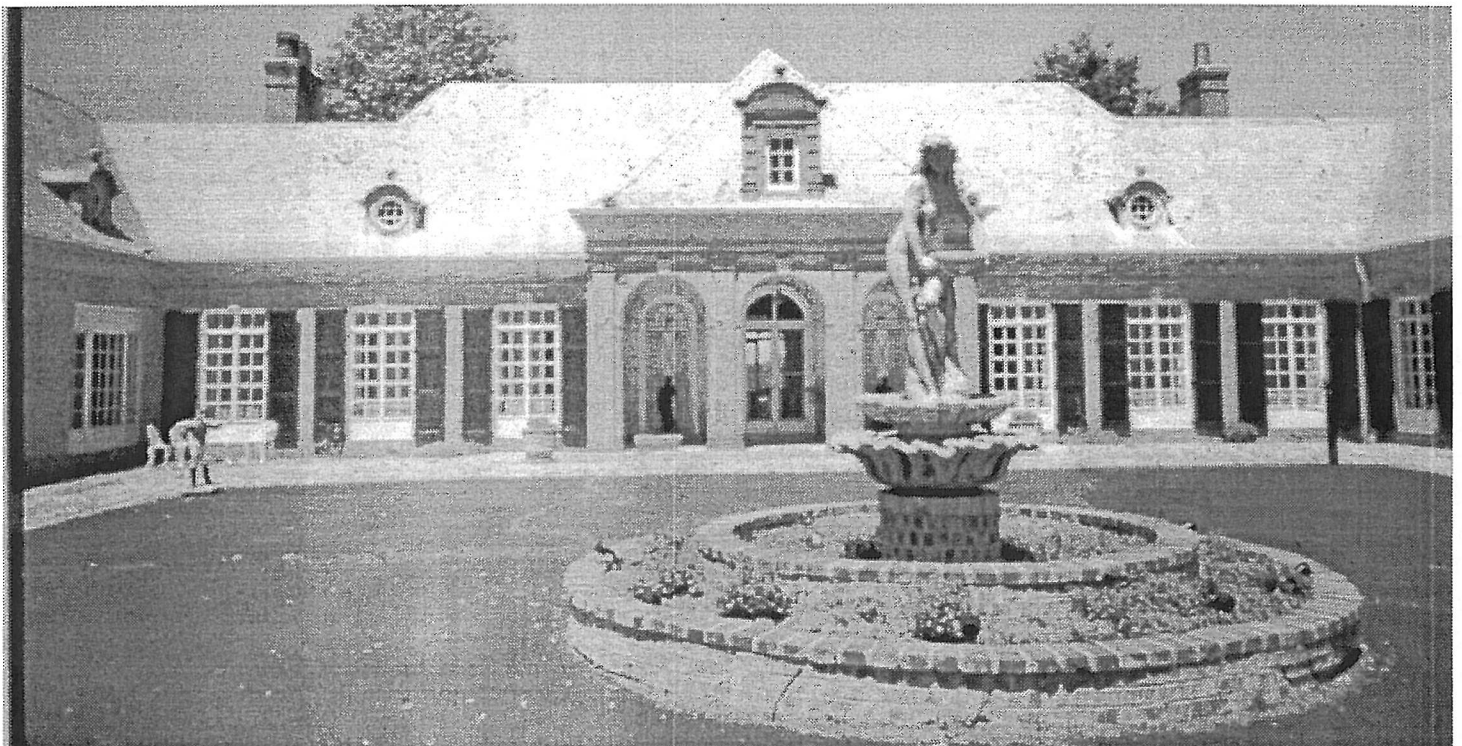
Entry of Mesker House, 1938. Photo by Daniel Williamson
