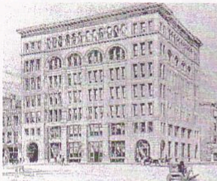
The Board of Education Building (called the Library on the picture) 901 Locust, Isaac Taylor, 1892
