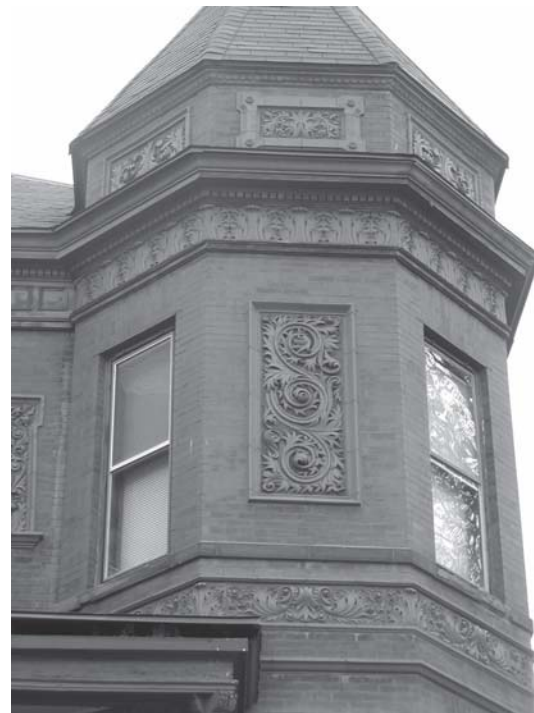
Herschel Bartlett Residence - 537 North 8 th Street
