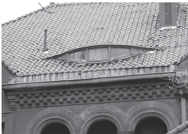
S. M. Nave Residence - 2121 Clay Street
