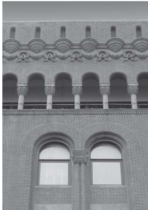
German-American Bank Building - 624 Felix Street
