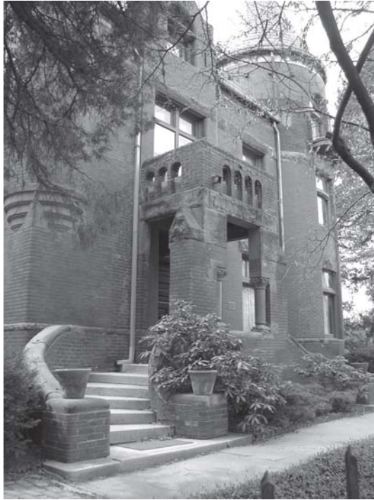
Alfred T. Smith Residence - 802 Hall Street
