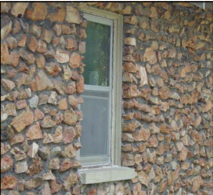
Figure Two —A Craftsman Bungalow built ca. 1930 at 2551 West High Street, with rubble walls, and dark gray mortar. The rock here is laid to create a highly textured surface. Rubble Construction
