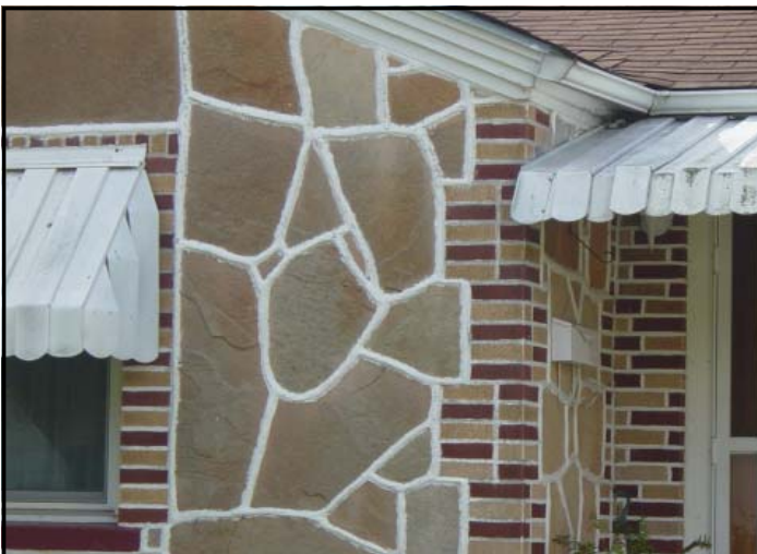
Figure Ten —Split Slab Construction
