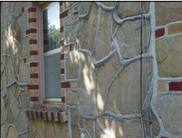
Figure Five —Skidmore house—split slab construction
