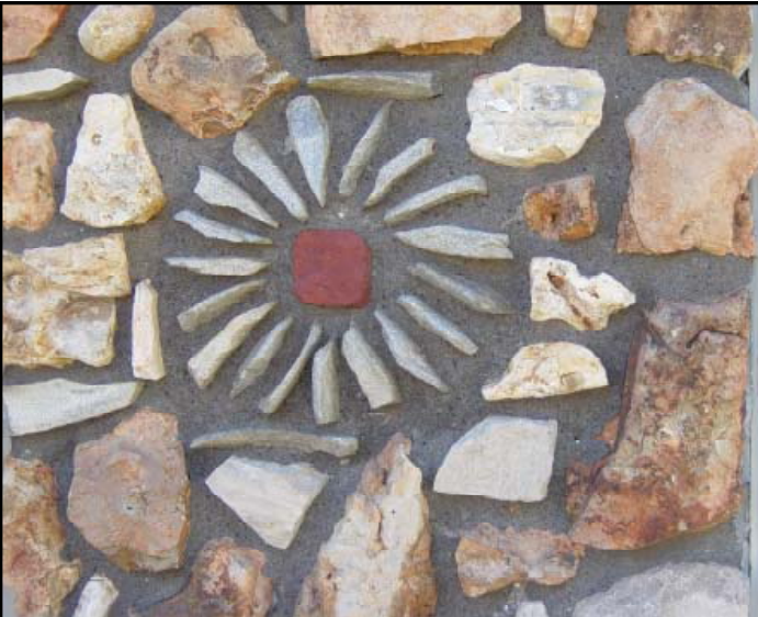
Figure Seven —Detail of Rockwork from the L. J. Kent Boiler and Sheet Iron Works, 700 E. Central Street, Springfield
