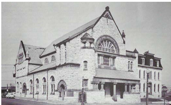
Temple Israel in 1960, HABS photo from Landmarks Association, St. Louis: Landmarks & Historic Districts, 1988, p. 50
