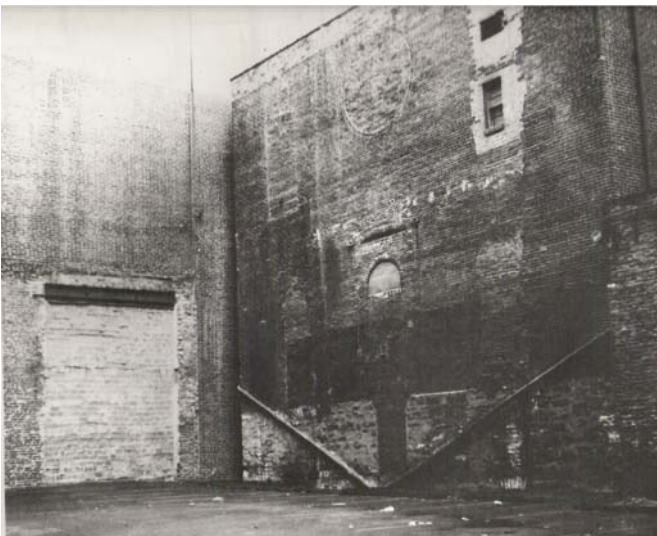
East wall of first United Hebrew in 1958. Note outline of rose window at top of wall. From Makovsky
