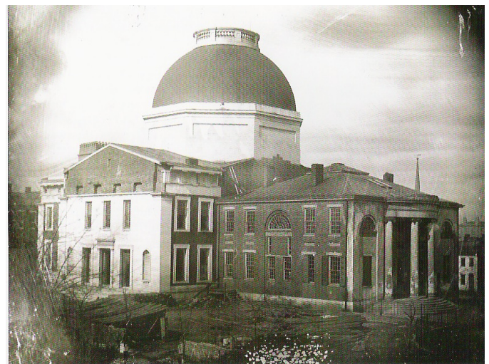
The Court House under construction in 1851, from a daguerrotype by Thomas Easterly. From van Ravenswaay, p. 326. The 1824 courthouse by Laveille & Morton was still standing on the right, and the original facade of the south wing (now an interior wall) remained as Singleton intended it to receive a Doric pediment and portico.
