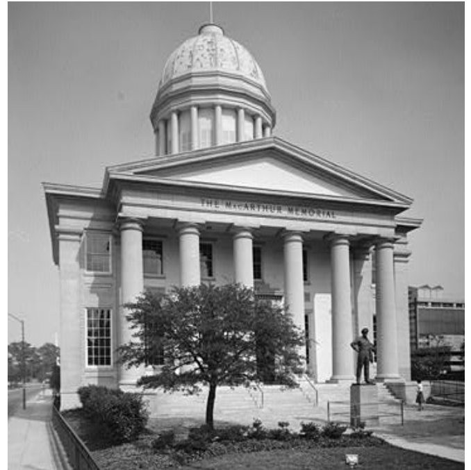
Norfolk City Hall, 421 East City Hall Avenue, Norfolk, Virginia, 1847-1850, William R. Singleton and Thomas U. Walter. HABS VA, 65-NORF, 10-1
