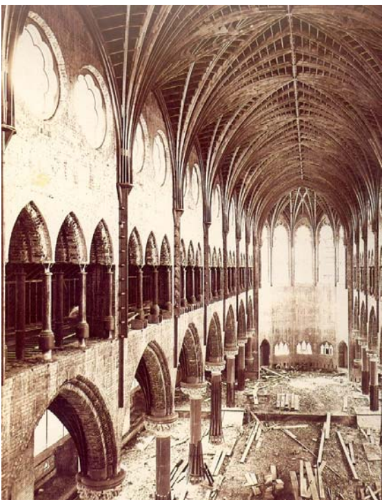
College Church under construction, showing the brick core of the walls and exposed lath of the vault webbing.
