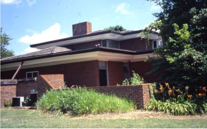
Malinmor, the southwest corner
