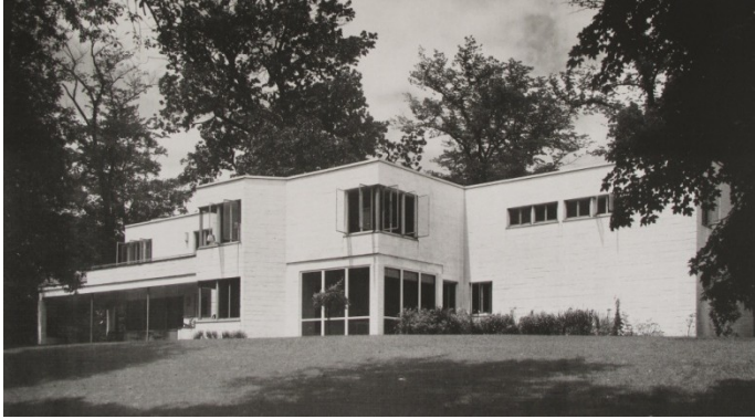
The Frederick & Harriet Rauh House, 10068 Leacrest Road, Woodlawn, Ohio, 1938, Garriott & Becker, garden front
