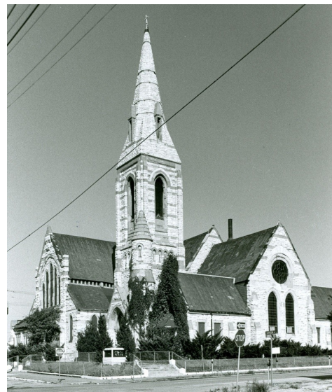
The earlier building of the Church of the Messiah, northeast corner of Locust and Garrison, 1879-1881, demolished 1987.
