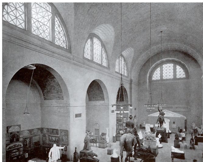
A view of the Great Hall of the St. Louis Art Museum before the Guastavino vaults were covered with a reinforced concrete shell
