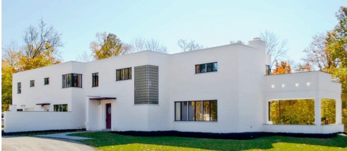
The Frederick & Harriet Rauh House, Woodlawn, Ohio, 1938, Garriott & Becker; entrance front, as restored
