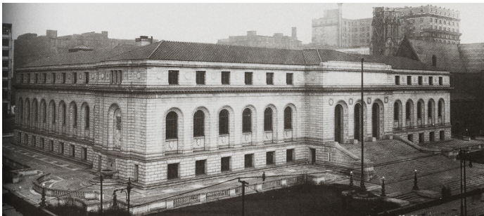
St. Louis Public Library, 1912, Cass Gilbert, a construction photo from Cass Gilbert collection at the New-York Historical Society
