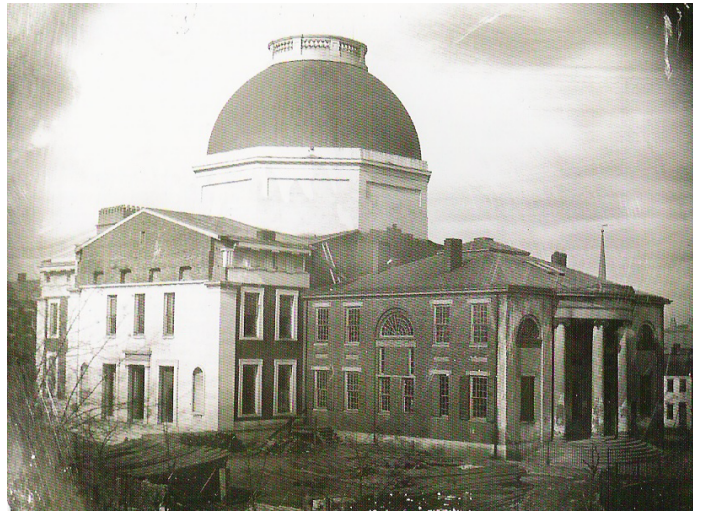
The daguerreotype by Emil Boehl dates from about 1851. It shows the 1828 Courthouse with the unfinished Henry Singleton building behind it. The south wing to the left was intended to have a pediment and portico, but instead an office wing was added by Robert S. Mitchell, and the Singleton dome was replaced by William Rumbold's iron one.
