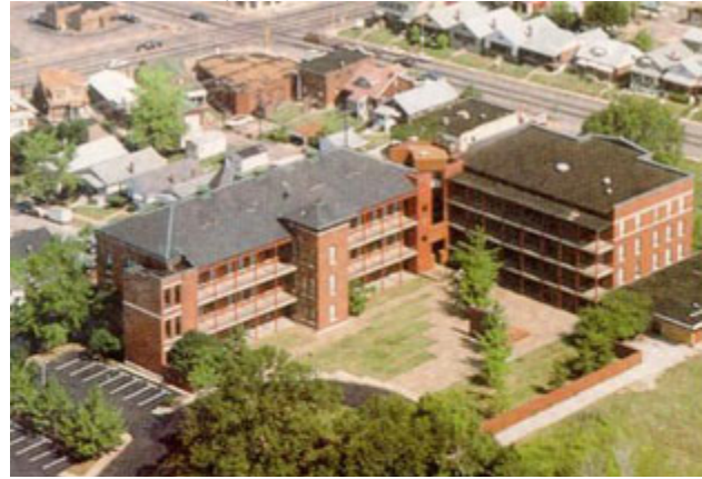
An aerial view of the only surviving parts of the Poor House complex looking northwest toward the intersection of Hampton (left) and Arsenal (right). The building at left appears on the 1903 Sanborn map while the one to the right is later, perhaps c. 1920. The two buildings were adapted as offices by the educational research laboratory CEMREL between 1970 and 1972. The Campbell Design Group bought the complex in 1985 and named it Campbell Plaza. This photo from CDGEngineers.com. shows the setting before the rest of the site was cut into a series of poorly planned residential developments.
