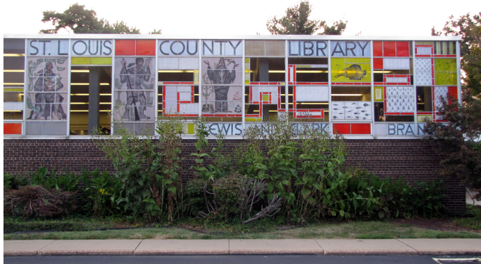
Exterior View, Main Facade, Northeast Corner, (photo by Lindsey Derrington)
