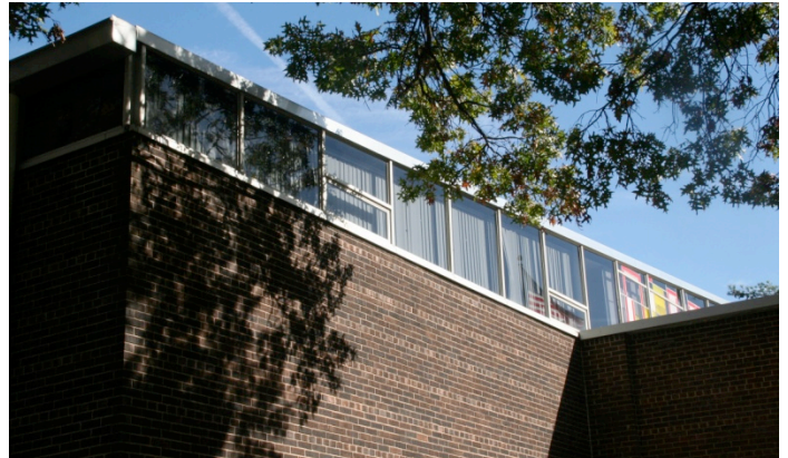
Southeast corner of library with clerestory (photo by John Guenther)
