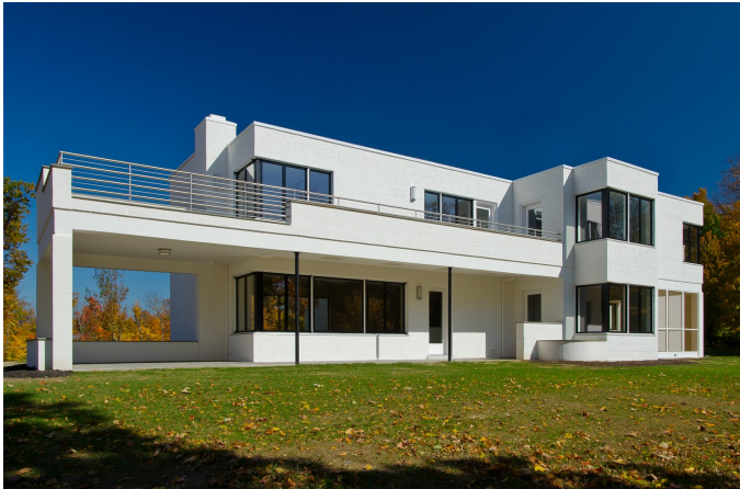
The Rauh House, Cincinnati, Ohio, 1938, John Becker, garden front
