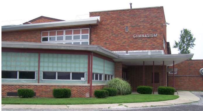
A corner of the gymnasium wing of Triad High School, Troy, Illinois, showing the light-directing glass blocks that were a critical part of the Maximlite concept
