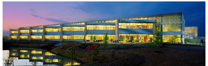
Alberici Headquarters, courtesy of Mackey Mitchell Architects Photo by Debbie Franke Photography, Inc.
