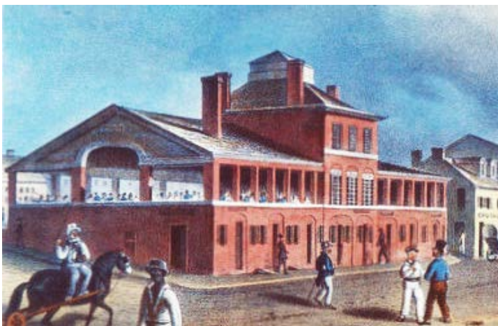
City Market and Town House, Front Street at Market St., shown in 1840 lithograph by J. C. Wild
