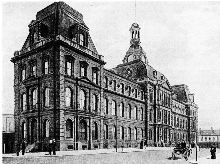
The Four Courts Building, from a c. 1900 postcard, Gateway Heritage, Winter 1999-2000, p. 13
