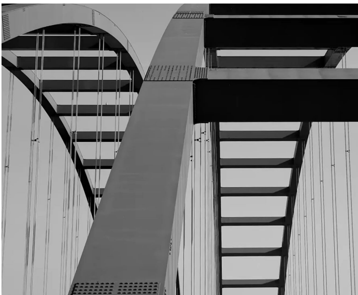
“Duo,” Jefferson Barracks Bridges, built 1982 & 1984, Alfred Benesch & Co. Photo by Ken Konchel. With spans of 909 feet, the bridges are the largest tied-arch bridges anywhere.
