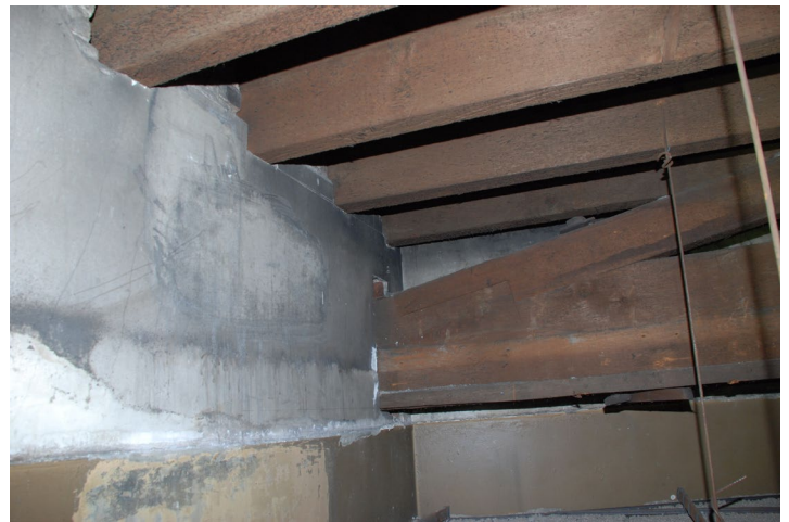
Wooden trusses and rafters in the Old Courthouse
