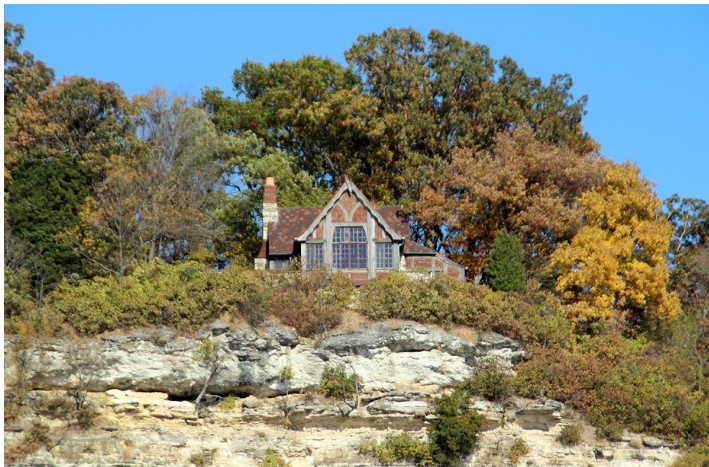
The Lodge, as seen from the Mississippi River, west of Alton (photo by John C. Guenther, FAIA, LEED AP)
