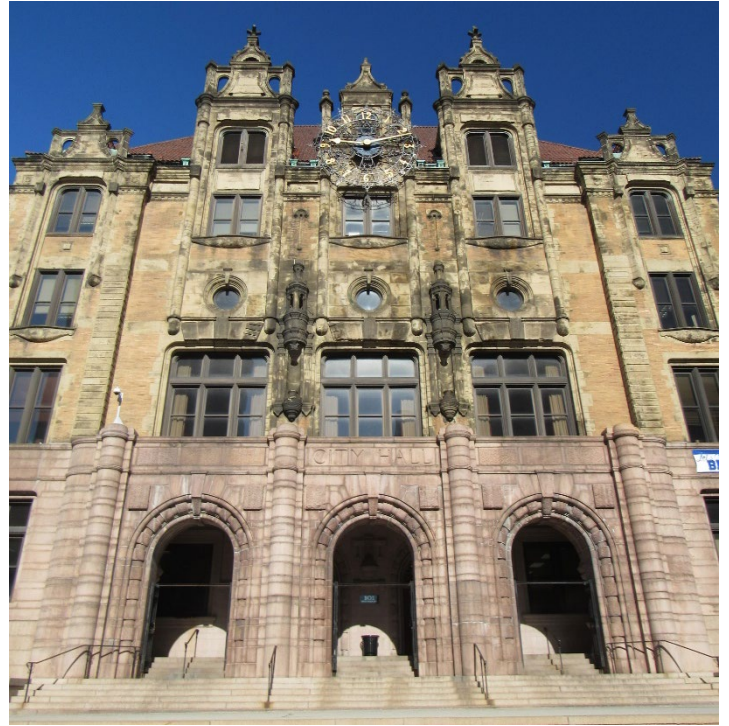
St. Louis City Hall, East Entrance photo by John C. Guenther, FAIA, LEED AP
