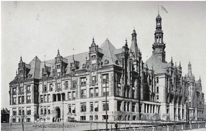
St. Louis City Hall Missouri's Contribution to American Architecture (1928) John Aubury Bryan, President St. Louis Architectural Club
