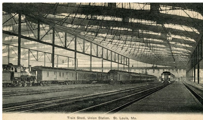
The Train Shed, designed by George H. Pegram, was the largest single-span train shed ever built, covering 32 tracks and over 12 acres with his patented truss.
