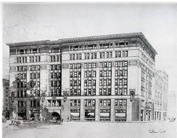
EDWARD MARTIN BUILDING, ST. LOUIS, MO. Geo. R. Mann, Architect.
