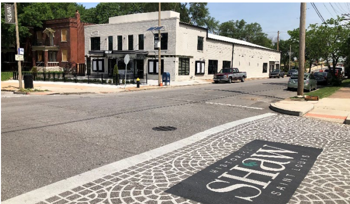
The historic Shaw Theater renovated into the Wild Carrot event space
