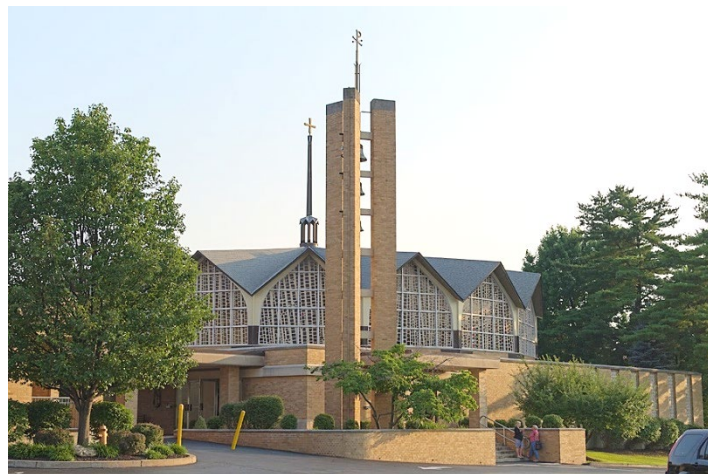
St. Clement Catholic Church (1965), 1508 Bopp Road photo by Mark Abeln
