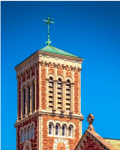
New pyramidal, low-slope standing seam copper roof minimizes the visibility of the roof, allowing for more emphasis on the cross raised high above. This roof also fits the Italianate style of the tower more than the original Victorian design. Photograph © Andrew Raimist.
