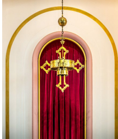
Chancel Chandelier hanging over the altar with electrical lighting hidden within the wider cylindrical element Eames inserted into the medieval Catholic original to accommodate this functional necessity. The position of this cylinder rests on the lower arms of the cross members and are thereby visible from the sanctuary. Photograph by Andrew Raimist for Eames Institute.
