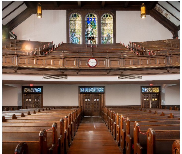
Three pairs of narthex doors with transoms at Pilgrim Church. Eames designed four new sets of doors with overhead transoms. The central set of doors are placed within a wider opening. Eames kept the doors the same size and inserted solid side panels. The fourth pair of narthex doors open onto the vestibule at the base of the tower to the north. Photograph by Andrew Raimist for Eames Institute.
