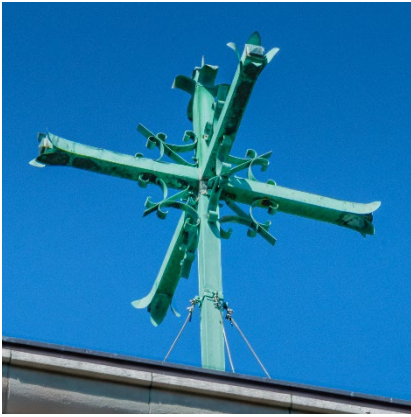
Charles Eames. New bronze and copper cross atop the tower. Note the flared ends of each member as indicated in the sketch as well as the thin diagonal members supported with scrollwork. Photograph © Andrew Raimist.
