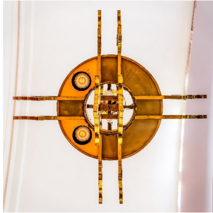
View of the Chancel Chandelier from below showing two recessed downlights at left surrounded by solid metal. The remainder of the donut-shape relies on glass with a metallic coating which offers diffused lighting. Photograph © Andrew Raimist.
