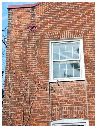
423 Miriam Avenue, east facade's brick masonry details.
