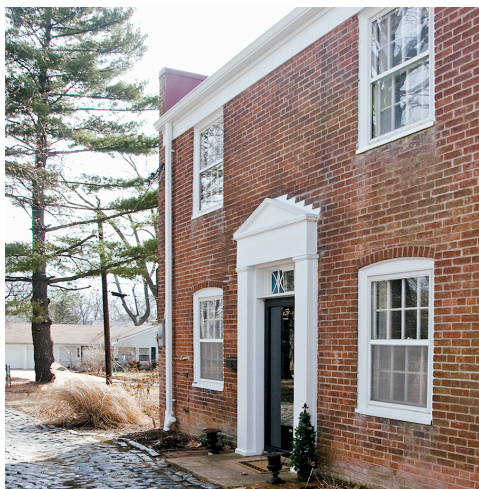
423 Miriam Avenue, Kirkwood, with entry facing north.
