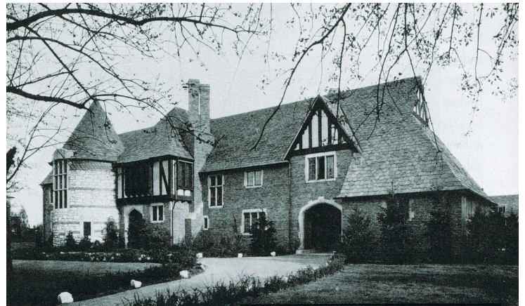
Maritz & Young, George Taylor House, 6352 Forsyth Blvd, 1926, now Washington University's Newman Center.
