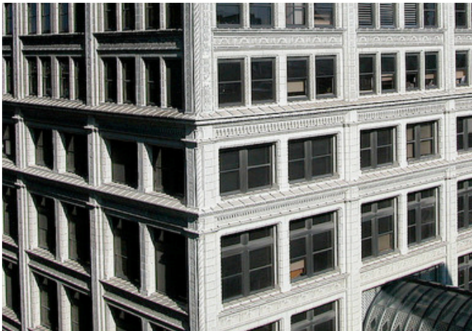
A detail of the Railway Exchange Building at 7 th and Olive, showing how the windows and terra cotta differentiate the department store floors from the offices above. Note how the string courses wrap around the corners of the 5 th and 6 th floors.
